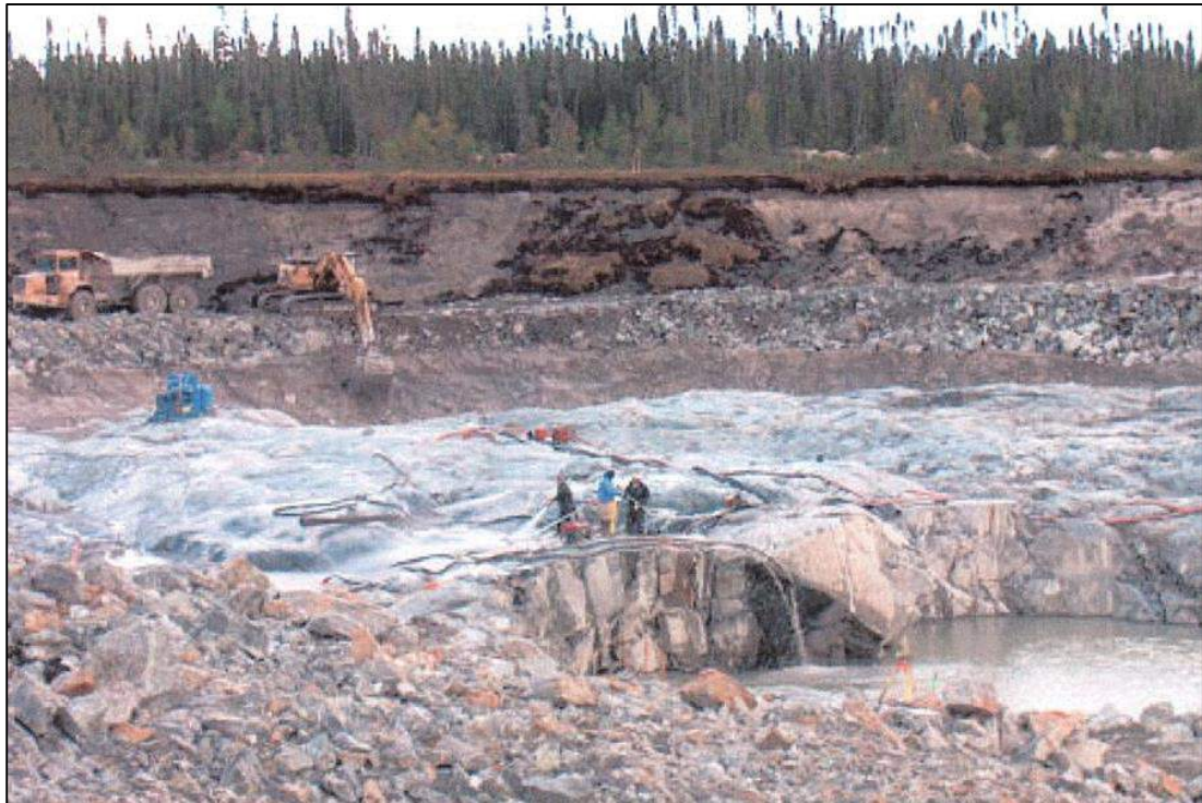
Figure 6.7 – Stripping work on the Discovery Zone (from Derosier, 2003)
